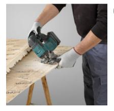
Place the panel in place on the wall where the corner is required. Draw a line down the back of the panel to mark where the mitre-joint will be cut. Using a circular saw or jigsaw cut the panel face-down at 45-degrees on the marked line.
