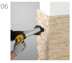
Once all the panels are in position fill any gaps, holes and screw holes with filler.
