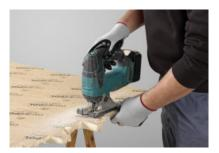
Using a circular saw or jigsaw cut the end of the panel to begin cladding the wall from one end.
