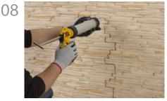
Fill the interlocking joints with filler for a seamless look. Also fill any screw holes where the panel is fixed.
