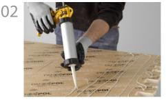
Apply adhesive to the back of the panel as a bead or blobs in a grid pattern.
