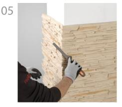
Fit adjacent panel forming a tight corner bond and fix the panel to the wall. If necessary smooth our any irregularities on the mitre-joint with a file.
