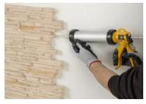
Ensure the interlocking fingers on each panel are glued to the wall.
