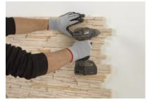
Screw through the panel to secure while the adhesive cures.
