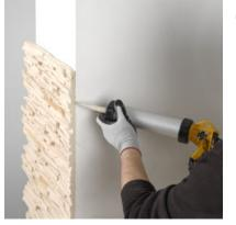
Apply adhesive bead onto the joint to glue both panels to each other.
