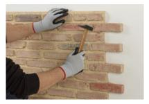
For masonary walls plastic expanding plugs and screws can be used to secure the panels.
