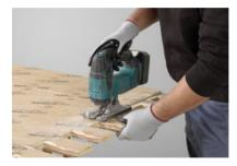
Using a circular saw or jigsaw cut the end of the panel to begin cladding the wall from one
