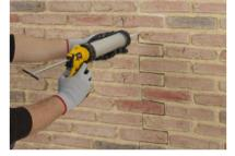
Fill the interlocking joints with filler for a seamless look. Also fill any screw holes where the panel is fixed.
