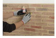
Let the filler dry for approximately 24 hours (depending on the temperature) and touch up joints and holes with correct colour paint using a small artist's brush.
