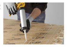
Apply adhesive to the back of the panel as a bead or blobs in a grid pattern.
