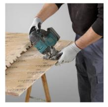
Place the panel in place on the wall where the corner is required. Draw a line down the back of the panel to mark where the mitre-joint will be cut. Using a circular saw or jigsaw cut the panel face-down at 45-degrees on the marked line.
