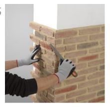
Fit adjacent panel forming a tight corner bond and fix the panel to the wall. If necessary smooth our any irregularities on the mitre-joint with a file.
