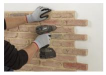
Screw through the panel to secure while the adhesive cures.
