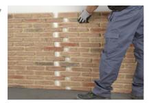
Place the next panel on the wall making sure the edge interlock fully seats.
